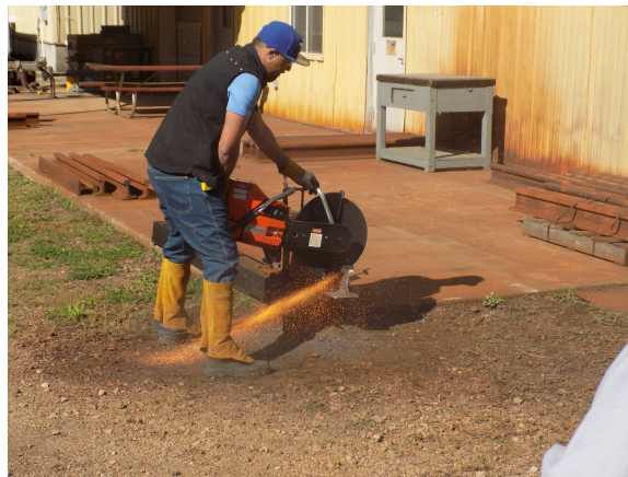
Rail cutting demonstration
